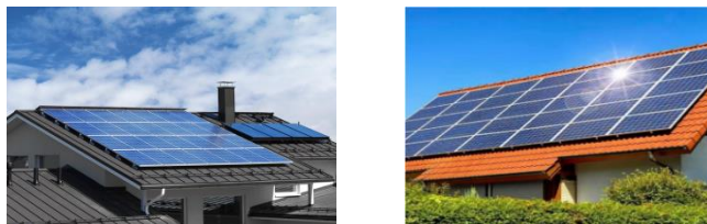
Figure 3. Installation of solar panels on the roof
